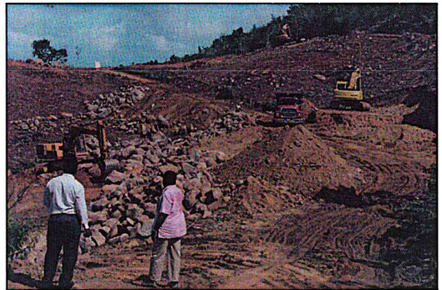
Contractor James Frett supervising excavation for HLSCC.
